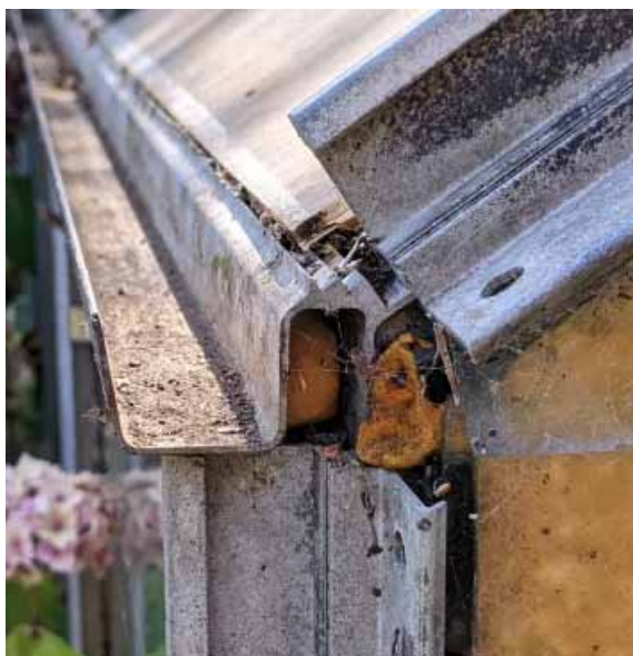
The gaps at the top of the vertical panels or glass where they meet the aluminium frame, now filled with foam
