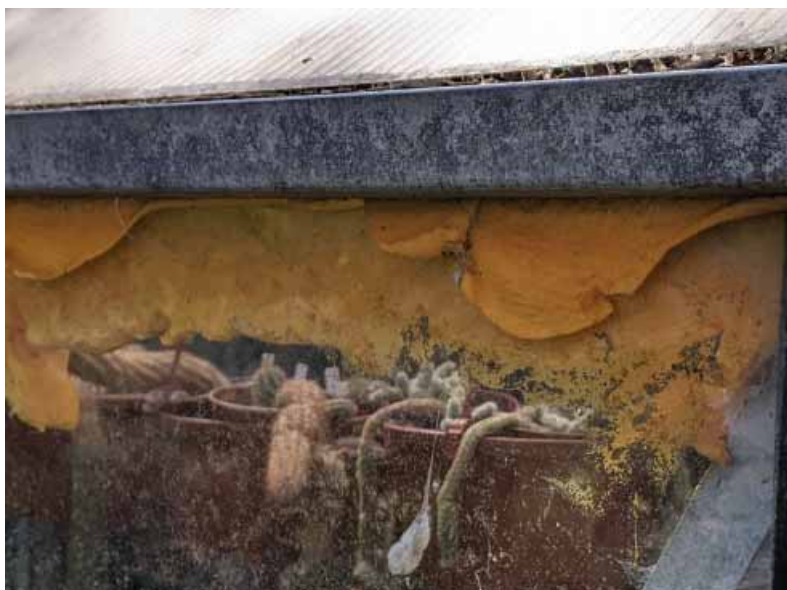
The gaps at the top of the vertical panels or glass where they meet the aluminium frame, now filled with foam
